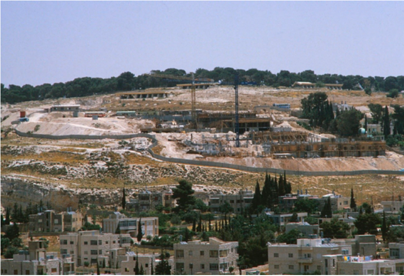
FIGURE 1. BYU Jerusalem Center under construction in June 1985. Photo courtesy Jeffrey R. Chadwick.
